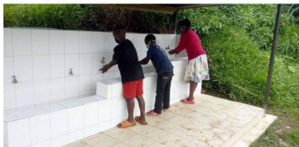
Hand washing station, fed from the school water harvesting system (August 2020)
